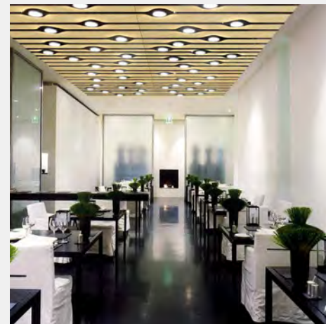
INLAY PLOT PANEL DIMENSION - 8'-0" X 4'-0" H PER PANEL MATERIAL - WOOD LIGHTING - LED
